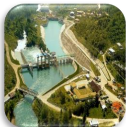
Poso Hydro Power Plant
