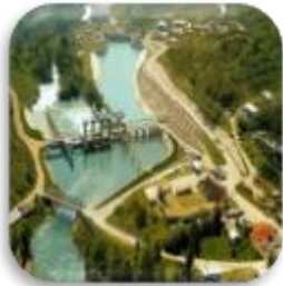
Poso Hydro Power Plant
