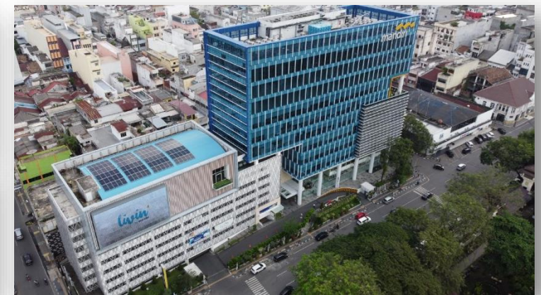
Solar Panels Implementation
